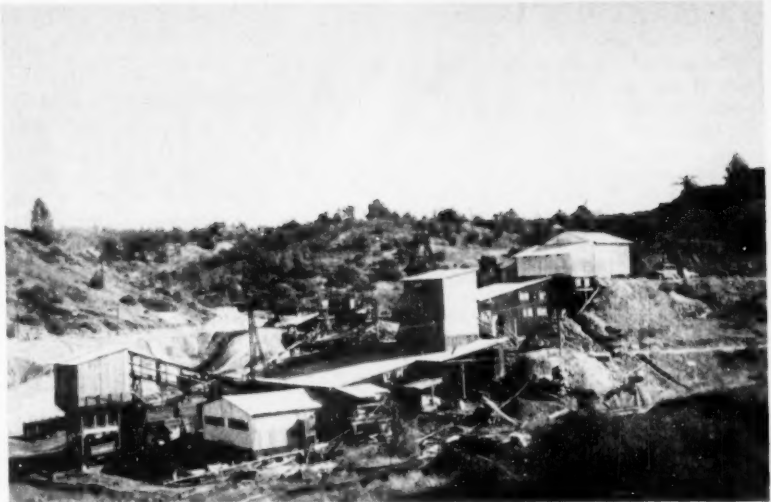
The old Penn mill has been reconditioned to produce gold amalgam and concentrates of copper-lead and zinc. It is shown here during extension of the near side to allow for future expansion to 200-ton capacity. The Penn No. 2 headframe can be seen above the center of the mill buildings.
